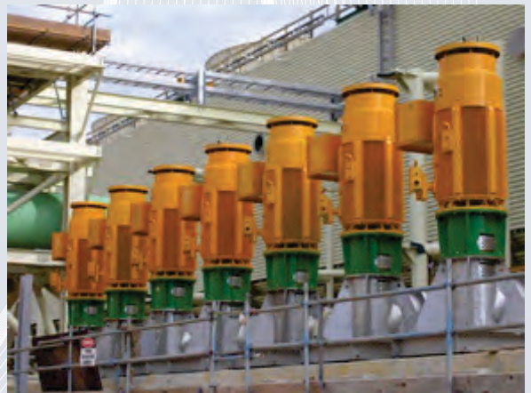
Duplex SS Seawater pump for Nickel Mine
